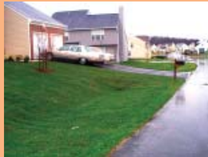
Grassed Swale and Street without Curb and Gutter
